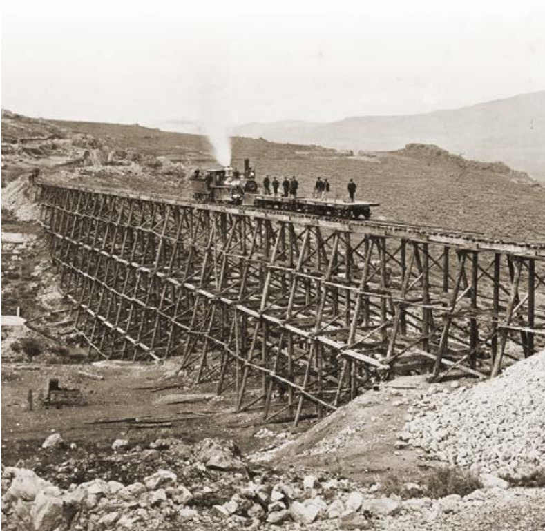
"Promontory Trestle Work and Engine No. 2", by Andrew J. Russell. This albumen silver print was taken in 1869. Russell chronicled the Union Pacific's east-to-west progress toward completion of the Transcontinental Railroad. Photo courtesy of the Union Pacific Railroad Museum.
